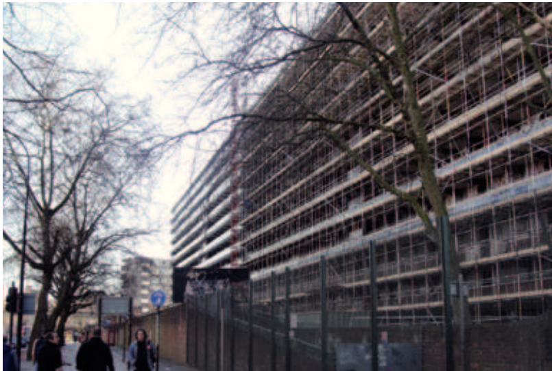
Photo 1: Heygate Estate completely empty awaiting demolition, 2014 (Photo: Lenimar Arends).
