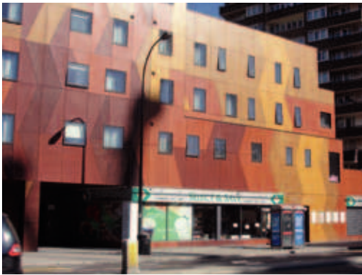
Photo 5: Building on Arch Street. Photography: Lenimar Arends, 2014.
