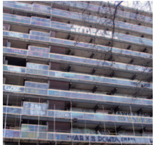
Photo 2: Heygate Estate completely empty awaiting demolition, 2014 (Photo: Lenimar Arends).
