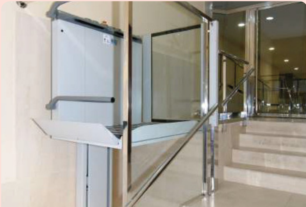
Renovated entrance hallway
