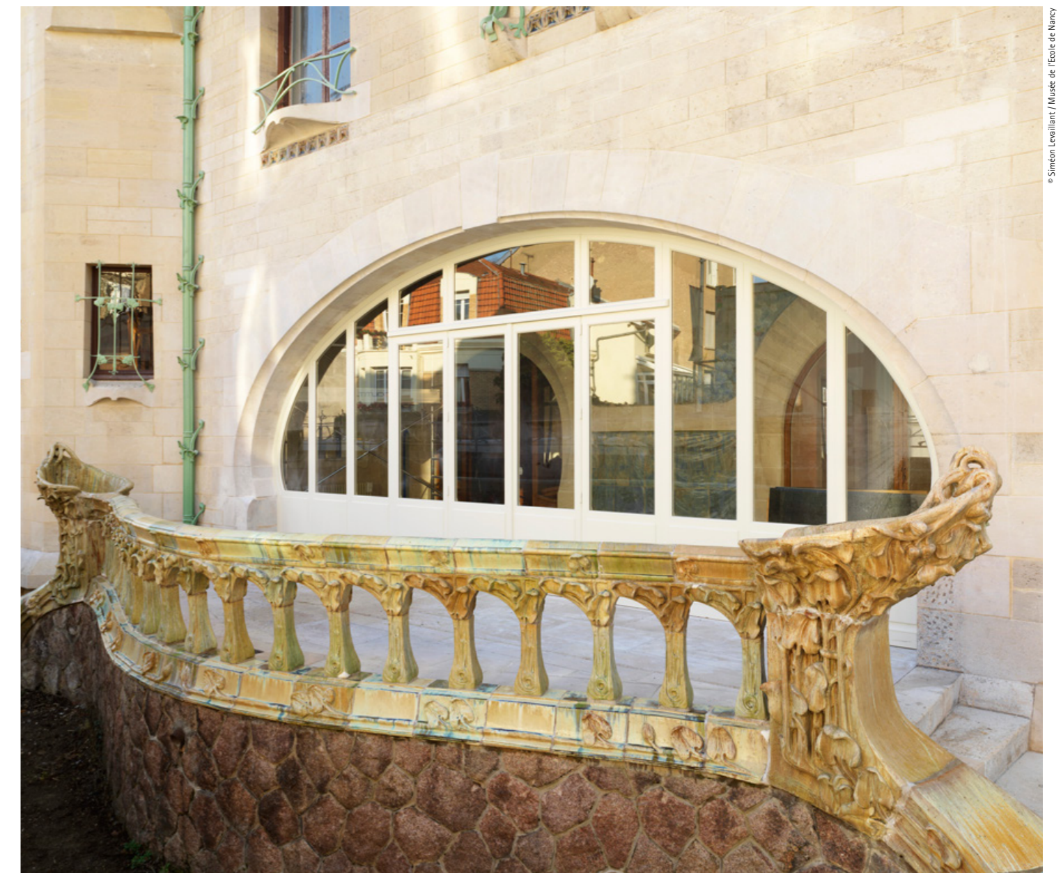
With the bay window removed, the terrace made by Bigot and Sauvage in 1907 was reconstructed to its original appearance Un cop enderrocada la tribuna, la terrassa construïda per Bigot i Sauvage al 1907 va ser retornada al seu aspecte original
