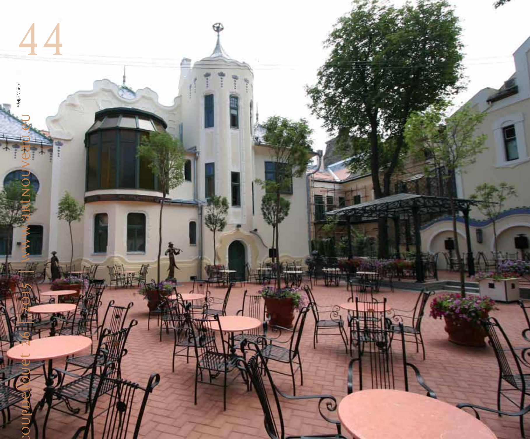
Present-day aspect of the rear façade and courtyard, with the new glass bow window that replaces the original one of glass prisms
