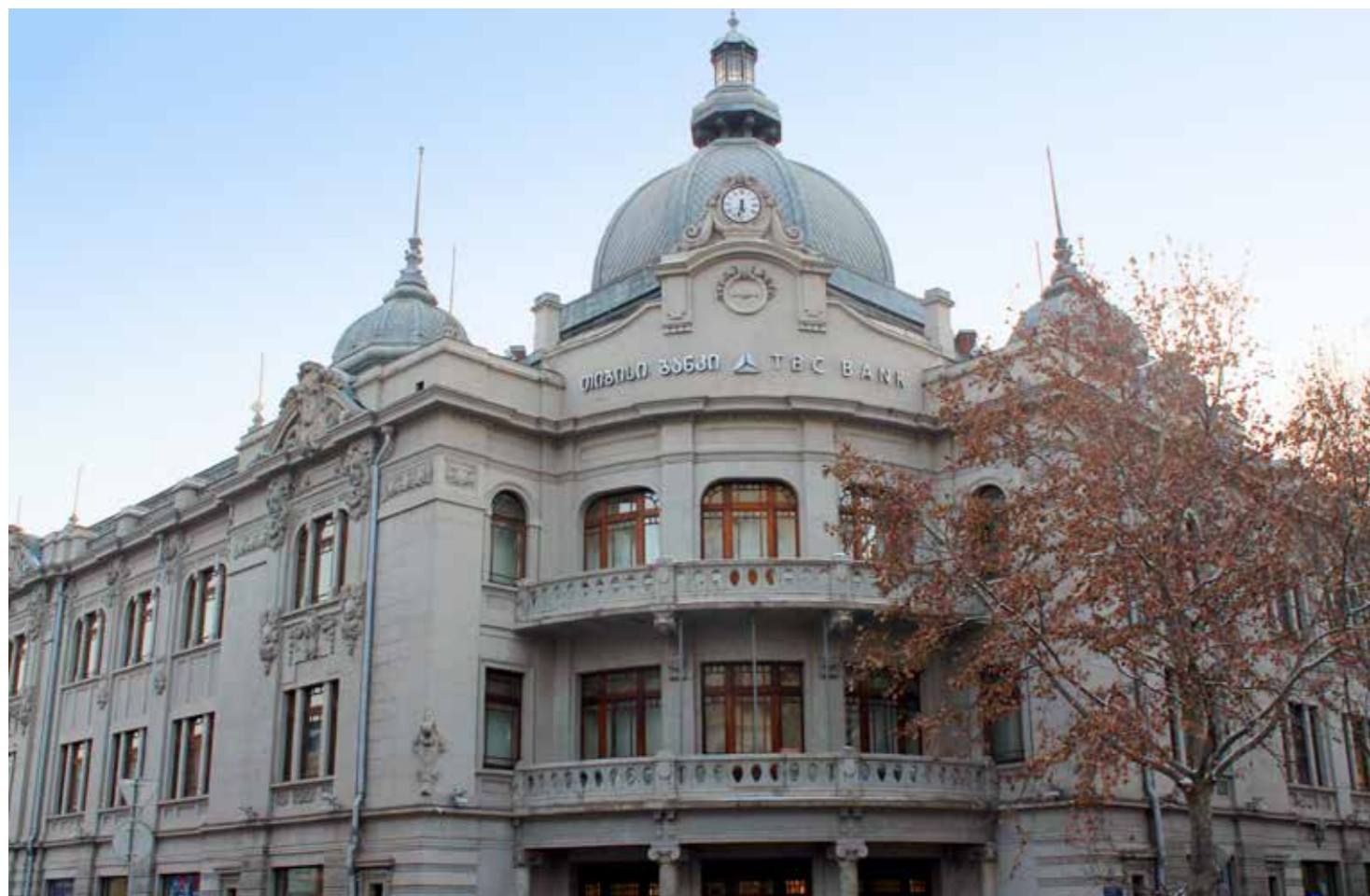
Present-day image of the central body of the building. The clock at the top was added during the last restoration in 2002. Under it, the 1920s cooperative symbol was preserved
