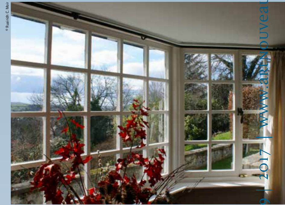
Canted bay window in the drawing room Finestral escairat a la sala d'estar
