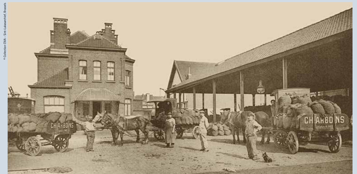
Victor Horta designed the central coal repository and foreman's quarters in 1899. Both buildings were demolished in 1988
