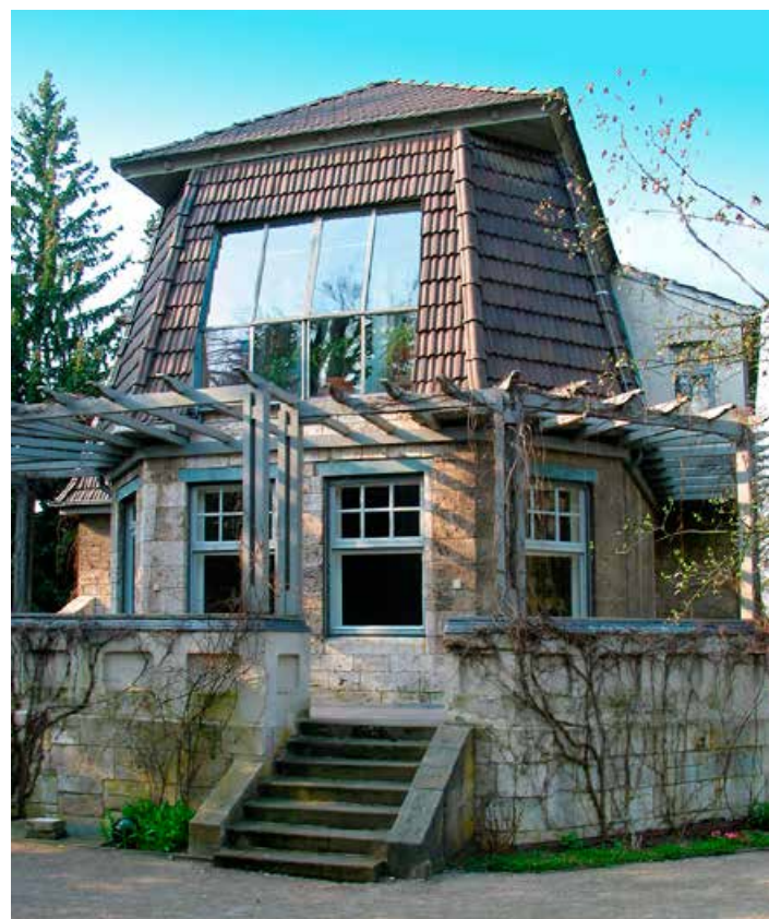
Henry van de Velde's house in Weimar (1907-1908). Photo taken during the association's excursion to this city
