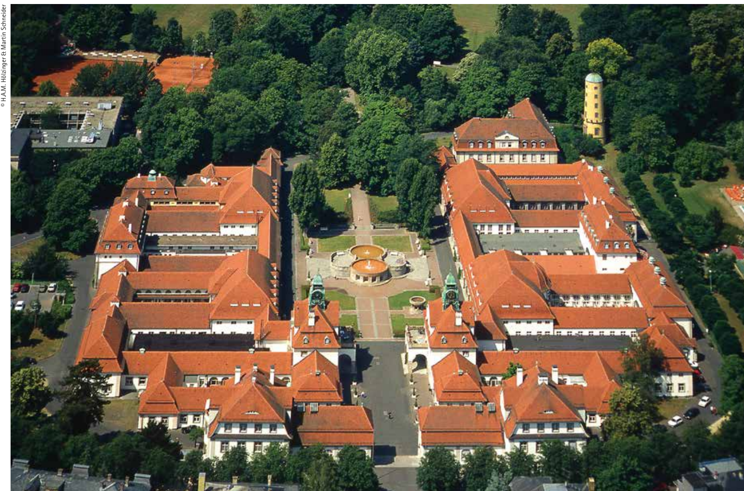
Aerial view of the Sprudelhof, the new spa complex designed by Wilhem Jost and built between 1905 and 1911
