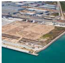
2 PRAT WHARF CONTAINER TERMINAL (PHASE 2) NON-CONCESSION AREA. MANOEUVRING AREA
