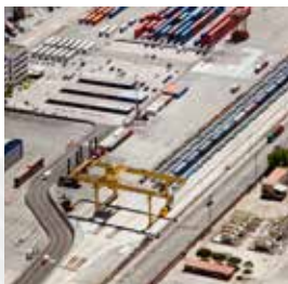
6 ENLARGEMENT OF THE SOUTH WHARF RAIL TERMINAL. PHASE II B
