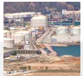
4 IMPROVED ROAD ACCESS TO THE ENLARGEMENT AREAS OF THE PRAT AND ENERGY WHARVES
