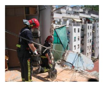
A home on the fifth floor of a building in Carrer Piquer was practically destroyed after a gas explosion on 5 May. The exact causes of the conflagration are not known, but it was triggered by a build-up of insecticide spray vapours that were trapped between the false ceiling and the terrace surfacing.
