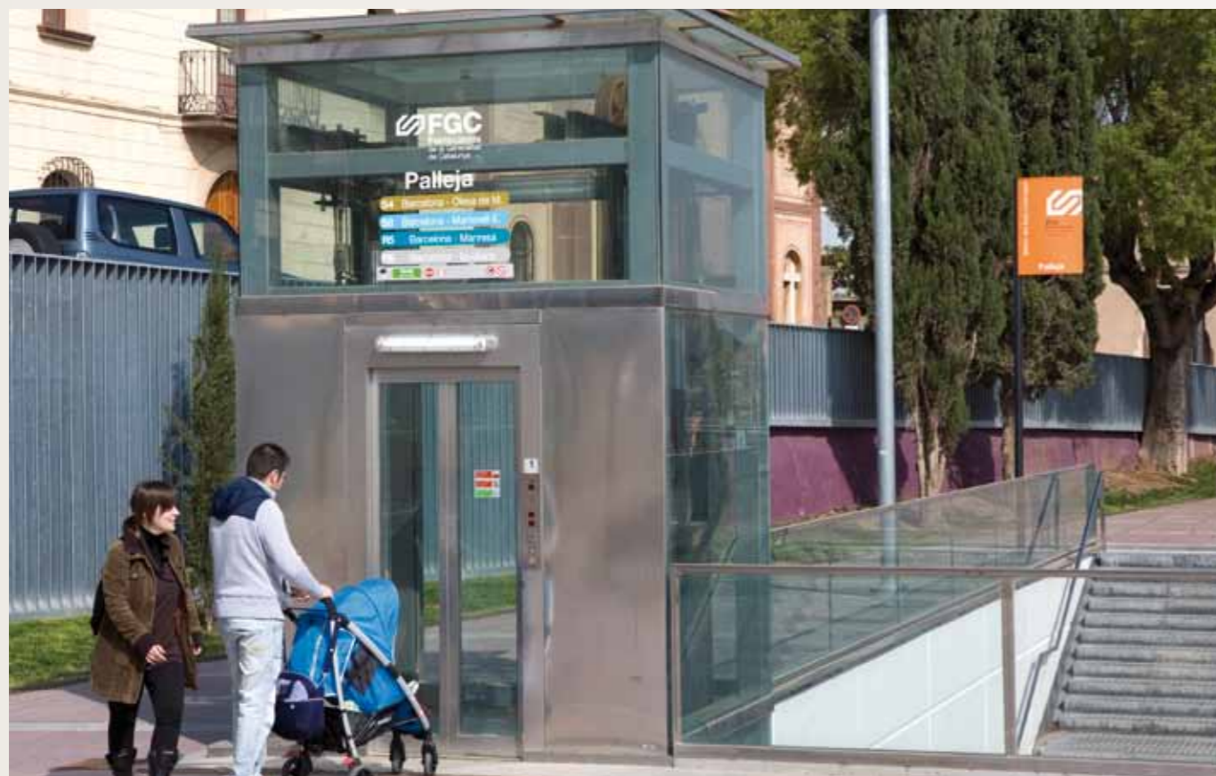
Pallejà. Lift at the Ferrocarrils de la Generalitat station.
