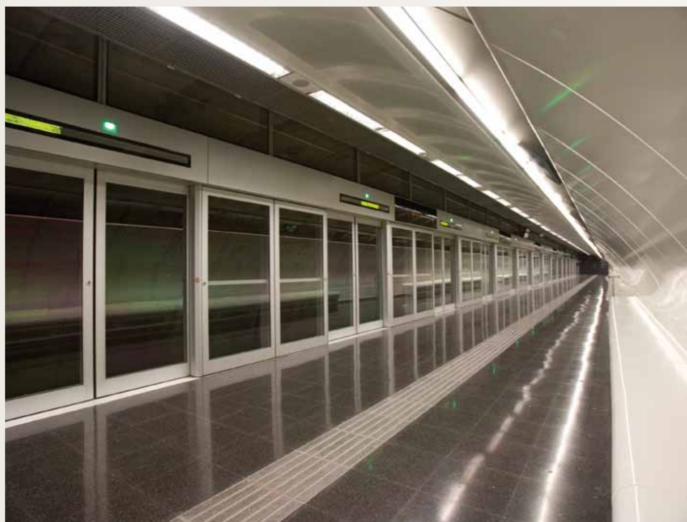
Metro line 9. Fondo station.
