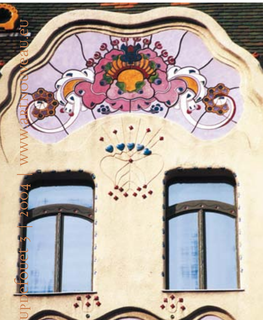
1910, Czifra Palota, Kecskemét, Hungary. Coloured tiles sunk into the plaster façade of the "Fancy Palace".
