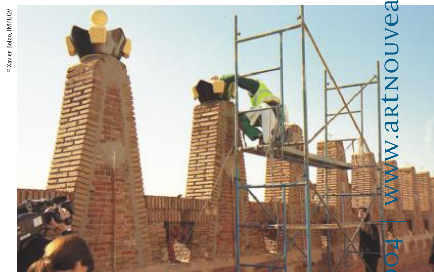
The birretas are reinstated / Els birrets es reposen.
