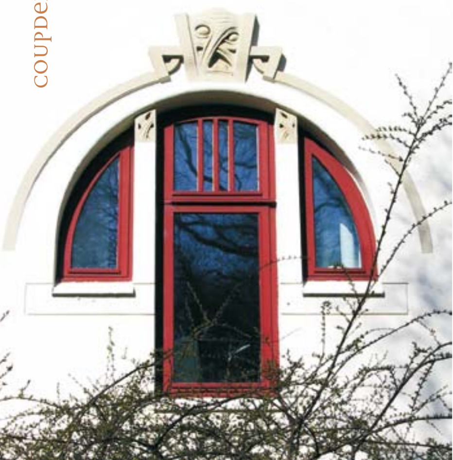
Schytte-Berg's ornaments were often sculpted by hand in mortar as part of the wall, as in this entrance to the Devold Villa
