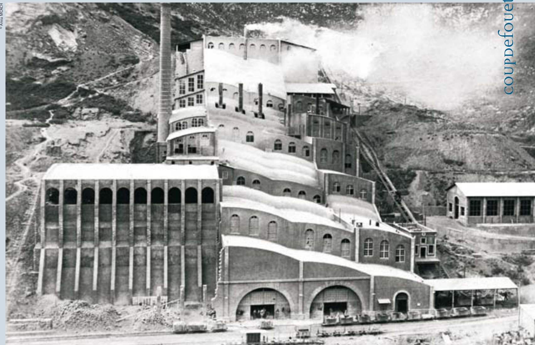
Former Clot del Moro Asland cement factory, in 1901
