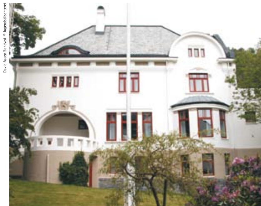
Devold Villa, 1905-1906, main façade
