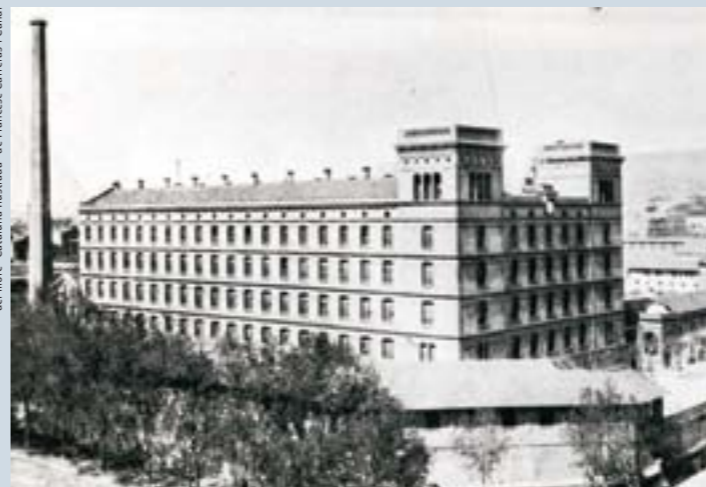
Former Batlló factory, 1869. General overview Antiga fàbrica Batlló, 1869. Vista general
