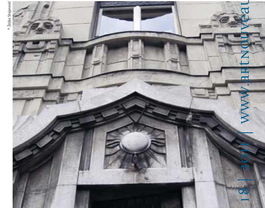
For the State Railways offices, architect Sandor Mezey imported popular Hungarian motifs in the façade decoration
