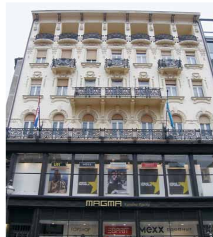
Hotel Royal building: Here, in 1906, Emilio Ambrosini applied concepts of Wagner's school for multi-purpose buildings, by combining a modern, sober structure of iron beams for the shop at the lower levels, with elaborate composition and decoration on the upper floors
