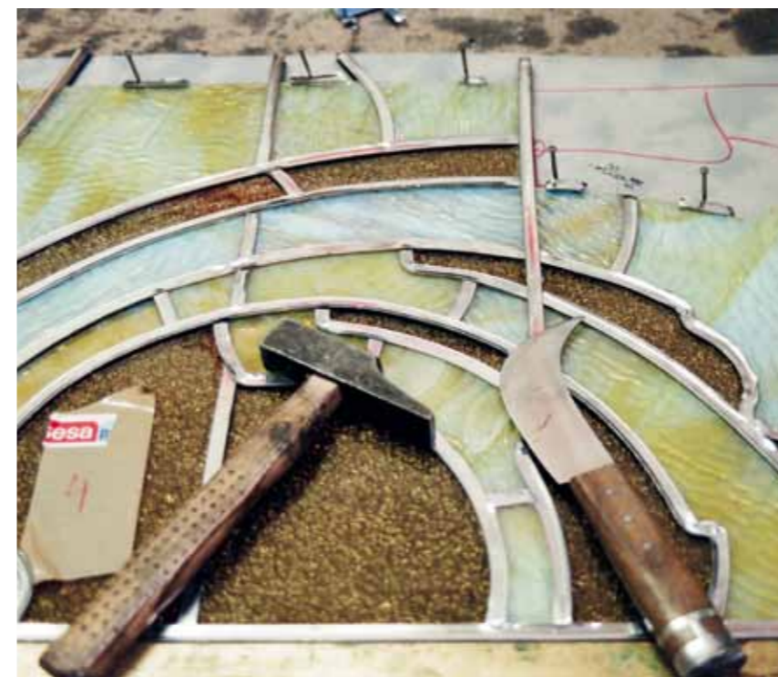
Detail of pieces from the main stairwell skylight during the restoration process
