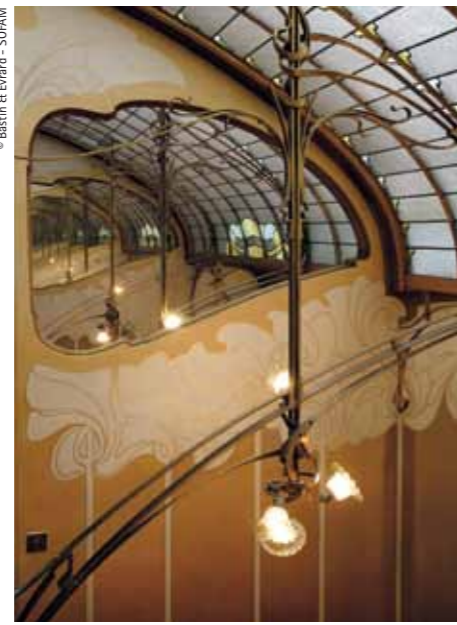
The main stairwell, complete with skylight and lamp, after restoration
