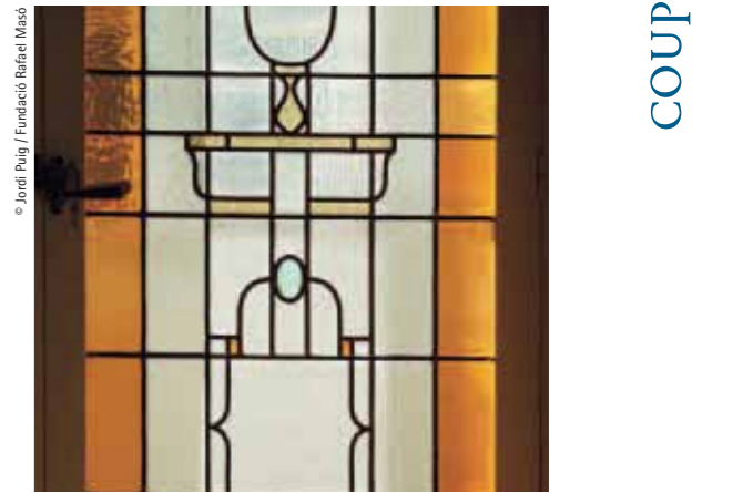
Casa Masó. Detail of a stained-glass window in a bathroom
