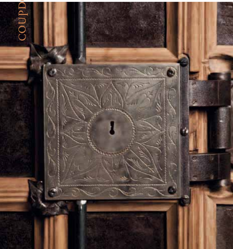
The painstaking restoration looked into the smallest details: lock of the door into Eusebi Güell's office
