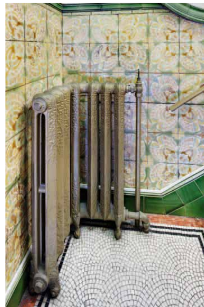
Original Art Nouveau tiles, mosaic floors and radiators are still preserved at the entrance area of the Miller and Lang publishing house
