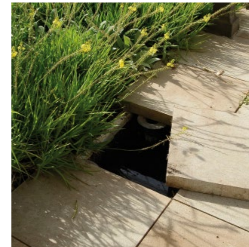
Detail of the cistern.
