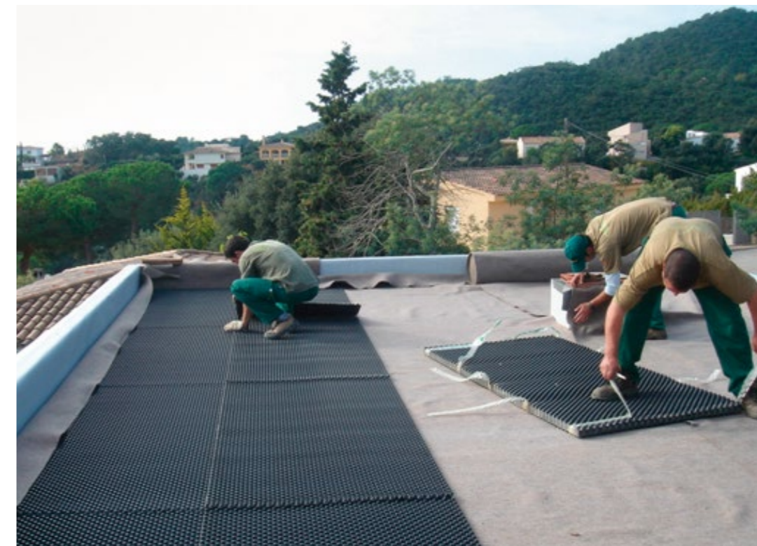
Installing a drainage board.
