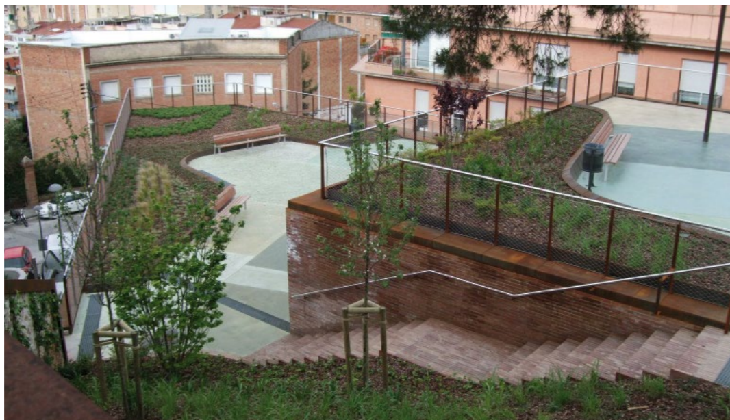
Building a green roof. Laguna Lanao Gardens.
